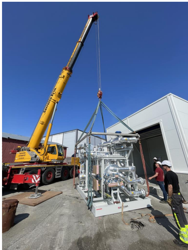
Figure 2. Mayekawa's Pentane heat pump being installed at Stella Polaris' site
